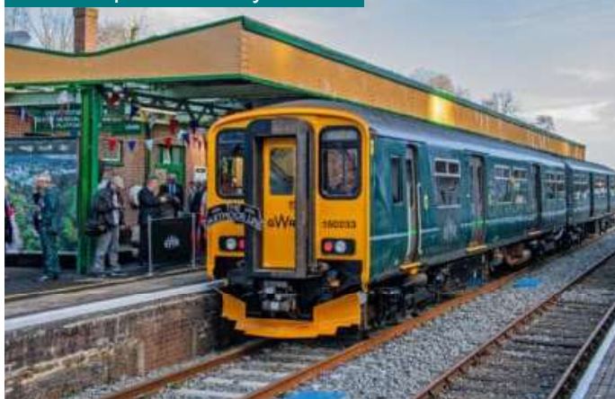
Okehampton Railway Station
